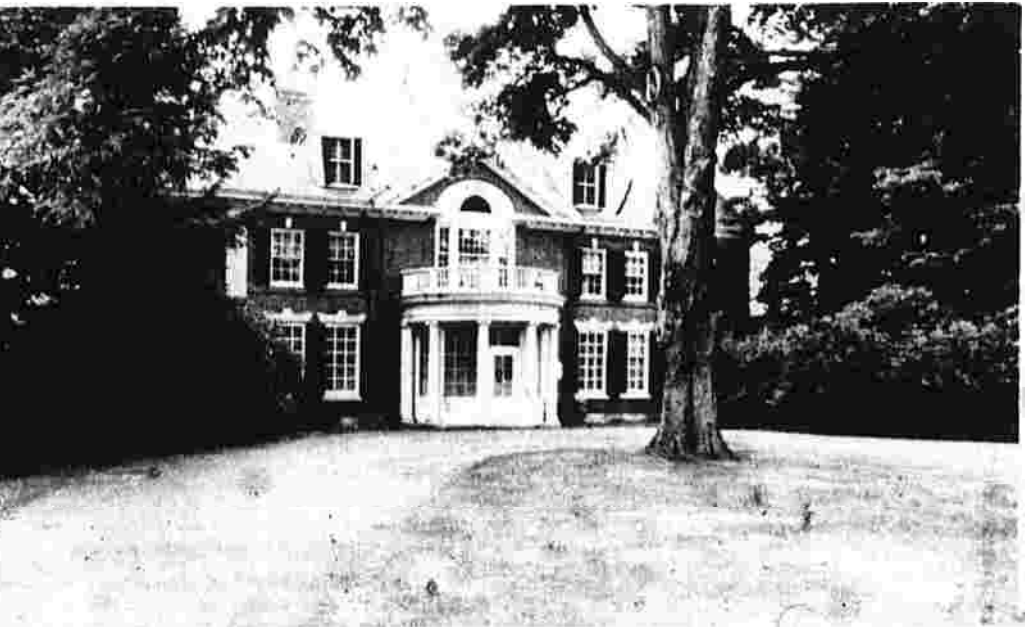
The South Methodist House at 20 Hartford Road, formerly the Frank Cheney Jr. home, was also designed by Charles Adams Platt and finished about 1900. This 2½-story, red brick dwelling sits on a stone foundation and has a hip-roofed central block adorned by massive red brick chimneys and simple banded dormers. Owned by the South Methodist Church it is used for both residential and assembly purposes. (Ofiara photo)
