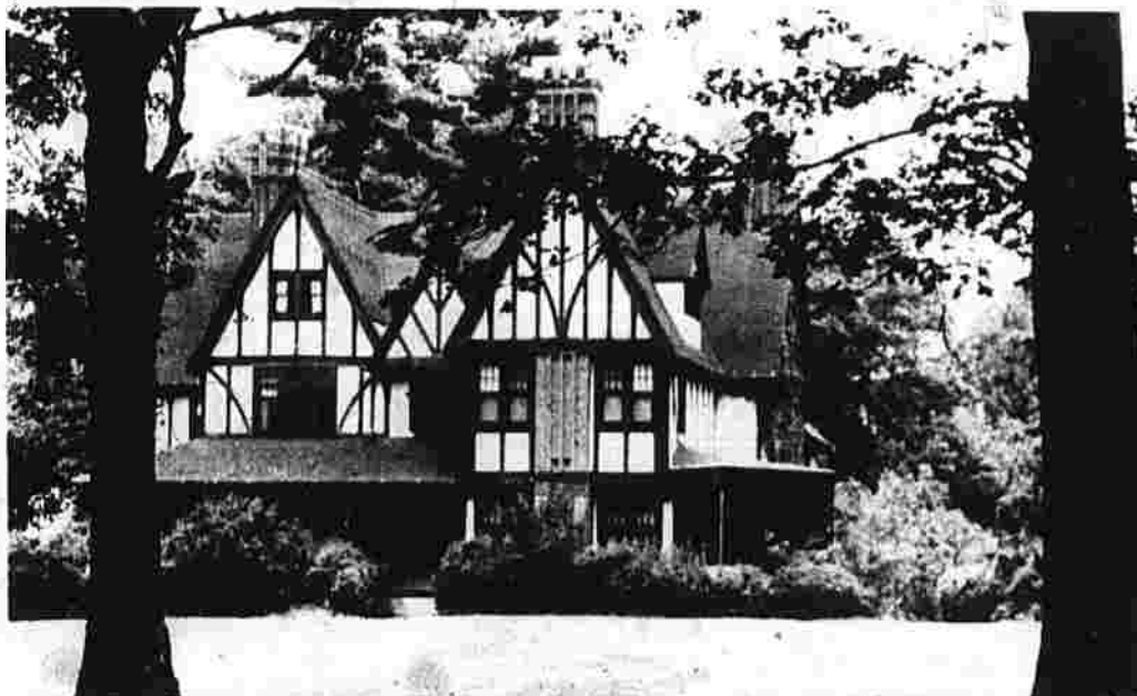
Built in 1880 as the home of Miss Mary Chapman, this dwelling at 75 Forest St., is the home of the Matthew M. Moriarty family. Originally, a wood frame structure, it was remodeled in the English Tudor-style during the 1960s after Miss Chapman's death. There is a total of 12 rooms and four baths and three large chimneys which allow for four fireplaces. (Ofiara photo)
